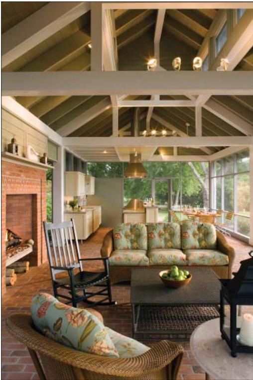
The screened porch was designed with an open plan. A roof monitor sits atop the room introducing light and air through serviceable windows. Structural rigidity and strength resides below the wood and brick surface in steel tube columns. This feature allows the near elimination of bracing walls on the perimeter. The brick materials in the floor and raised plinth were carefully selected to resemble the brick used in the foundation of the original house.
