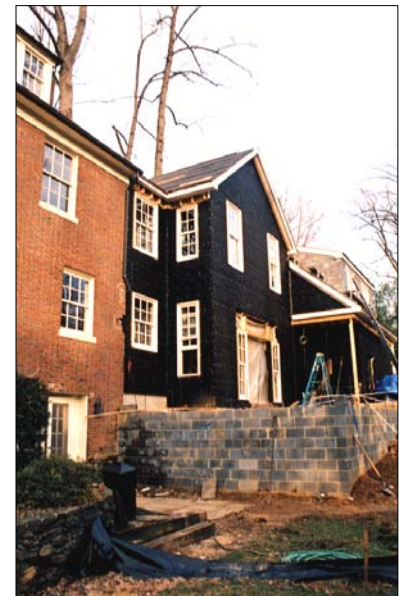
RETAINING WALL FOR NEW TERRACE UNDER CONSTRUCTION
