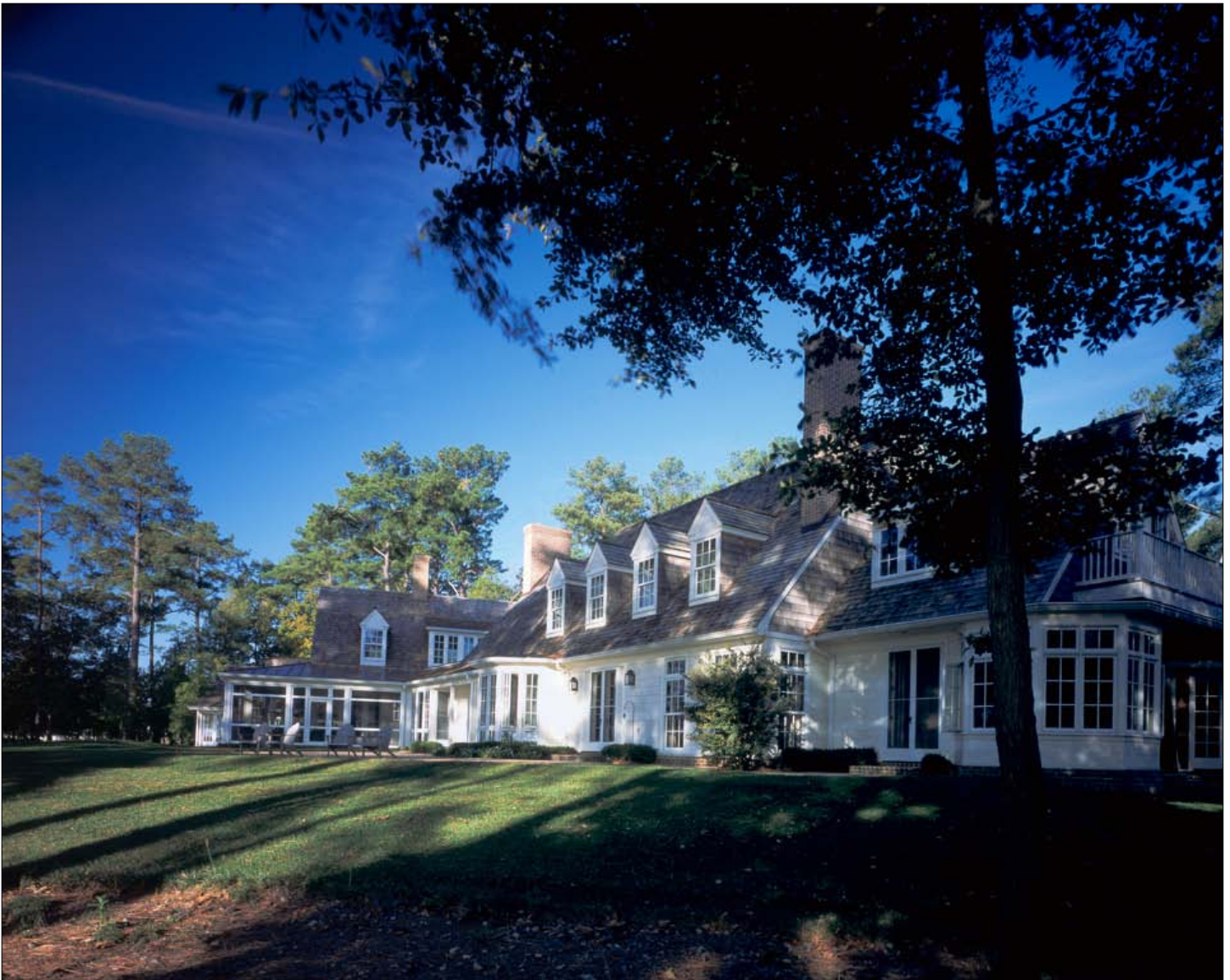
BELOW: THE FULL ELEVATION OF THE WATER SIDE OF THE HOUSE.
