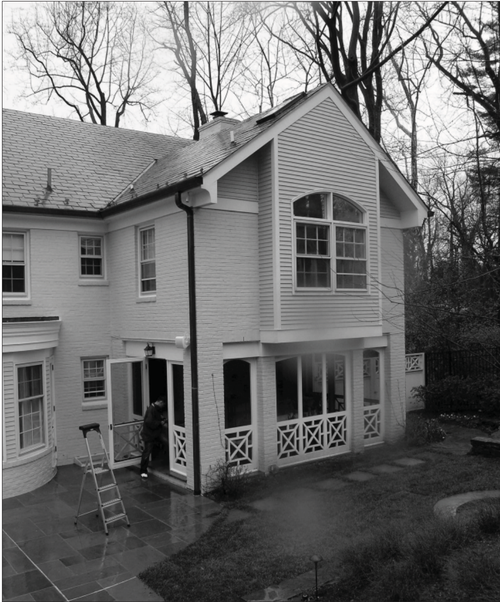
Rear Elevation, Before
